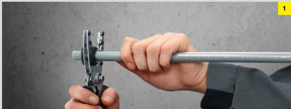
Cut pipe to length using the Raxinox pipe shears.
