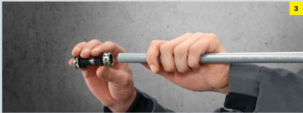
Position the connector. Check insertion depth in the inspection window.
